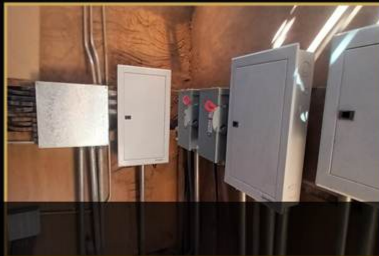
ENGEX ELECTRICAL INSTALLATION
