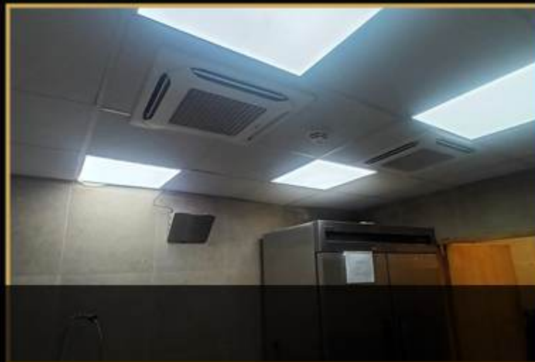
REAL ENGEX HVAC INSTALLATIONS
